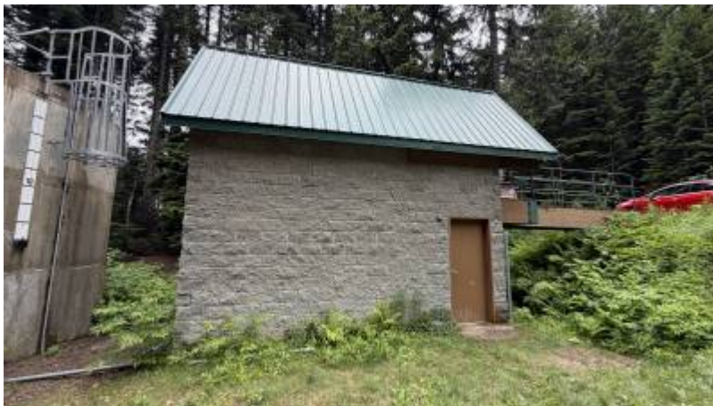
Figure 2: The side of the pump house and ground floor door.
